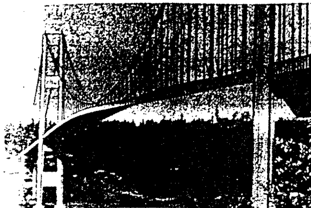
Fig. 1. The original Tacoma Narrows bridge under the action of wind. 1
